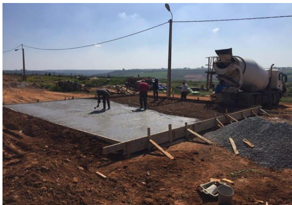
Figure 1. Photography of platform under construction
